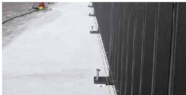
Assembling of supporting props
